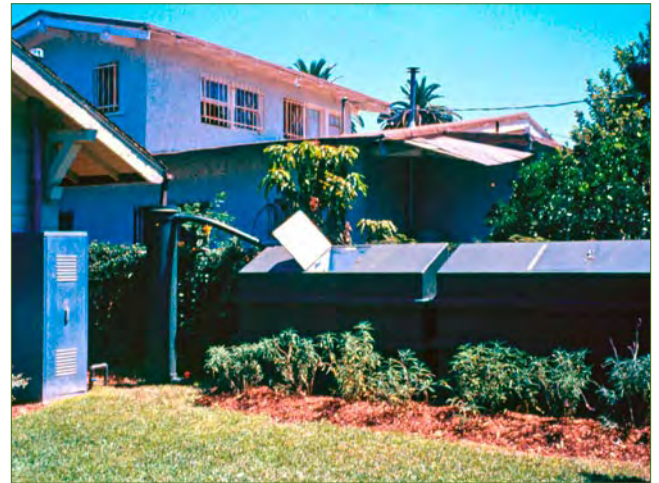
The cistern system captures stormwater falling on a portion of the roof. Together, the cistern's two recycled plastic tanks provide 3,600 gallons of storage space. A pump distributes water to the irrigation system.
