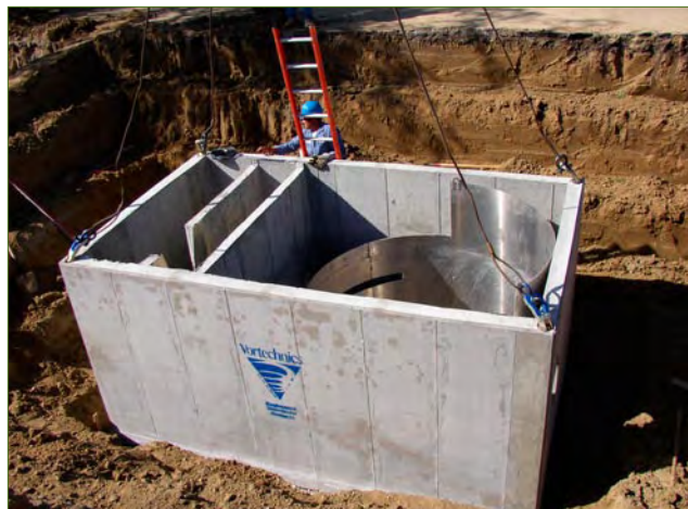
The Vortechs 7000 treatment system uses swirl technology and gravity to separate and retain pollutants, oils and trash from stormwater.
