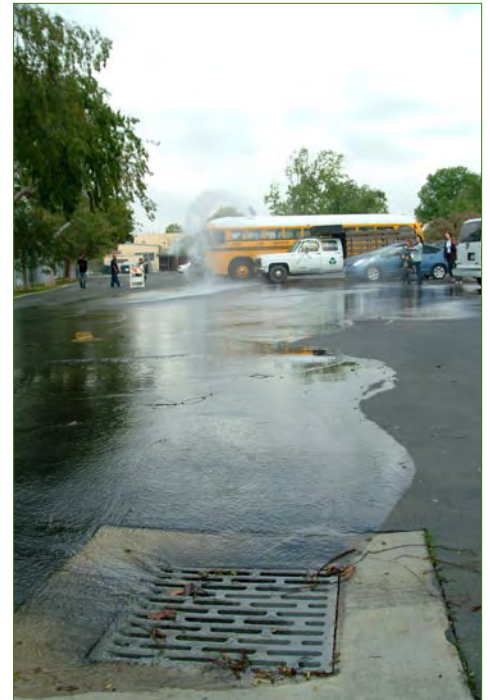
Water drains into a storm drain after a mock flash flood at Open Charter. Rather than running off the campus and eventually into Santa Monica Bay, stormwater is collected and detained onsite by a system of BMPs including trees, vegetation, swales and a cistern.
